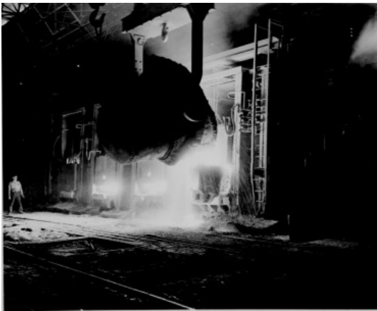
1/ JONES AND LAUGHLIN STEEL COMPANY, PITTSBURGH, MAY 1942
