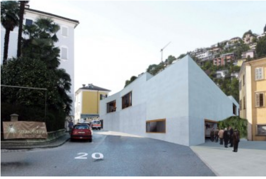
PROJECT BY LUKAS GERMANN: EXTERIOR VIEW.
